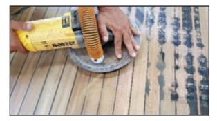
**16.** When caulking has cured, sand surface of deck to remove excess caulking using 80-100 grit sandpaper with a soft pad on a grinder.
