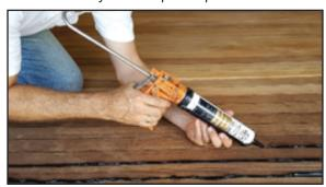
13. Ensure caulking goes to bottom of seam, allowing it to flow upward until crowning above the top of the seam. Smoothly pull the gun along the seam toward the applicator. Avoid starts & stops or changes in direction that may entrap air. NOTE: If using pneumatic caulk gun do not exceed 80psi to prevent overriding the plunger and injecting air into the caulk.
