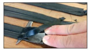
15. Allow caulking to cure for at least 48 hours (longer in cold weather and for larger seams). White and grey caulking need at least 8 to 12 days to fully cure. See "White & Gray Caulking" section for more detail. Removal of excess caulking can be done by Fein tool or sharp chisel.
