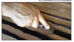
14. Immediately after application, draw a flexible putty knife over the seam at a 30° angle. Apply enough pressure to make sure caulking fills to bottom of seam, but leave the caulk high to allow for slight settling. Make sure seam has no entrapped air after application. Do not disturb until fully cured.
