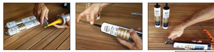
**12.** Cut the tip at a slight angle with a razorblade. Insert sausage or cartridge into gun.
