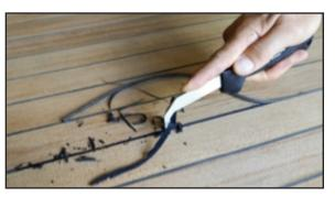
2. Reefing hook scrapes out caulk sealants once they have been freed using a razor knife. It leaves minimal material residue, so the seam can be easily sanded.
